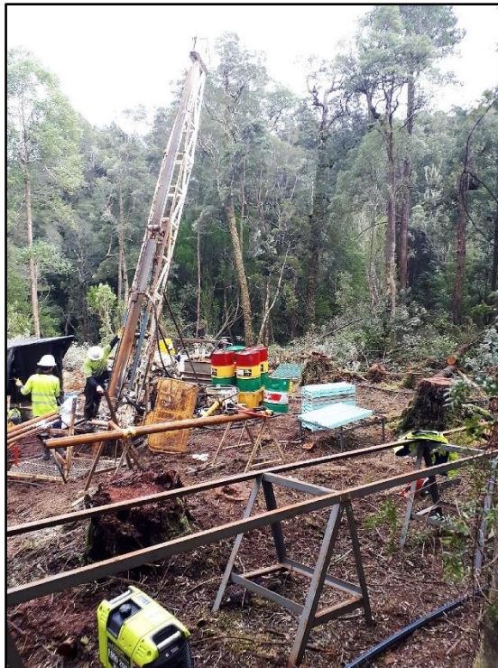
Photo 1: YHDD001 drill rig on site
